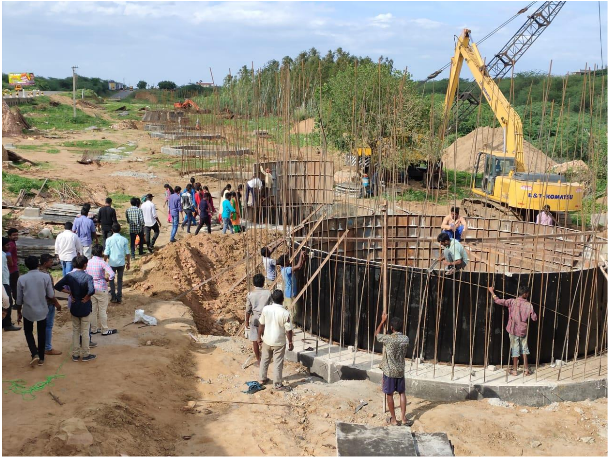
Students observing various components of Bridge.
